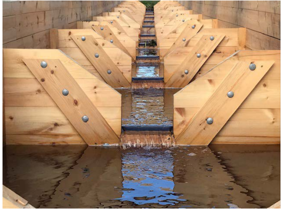
Figure 59. The old fish pass is removed (upper left) and the new one is installed. When the leak was sealed all pools was filled as planned (lower right). Photo: Oliver Karlöf.
