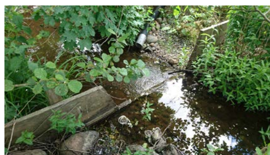
b. Wooden threshold downstream of the fish pass, Migration obstacle at low flow conditions.
