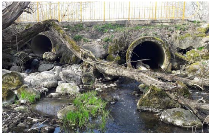
Figure 33. The two culverts that constitute migration obstacles.
