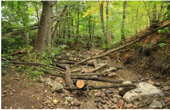
Figure 45. A mixture of gravel, larger stones and existing logs were placed on stretch 1 and 2. Photo credit: John Kärki.
