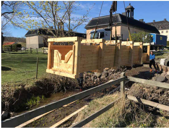
Figure 59. The old fish pass is removed (upper left) and the new one is installed. When the leak was sealed all pools was filled as planned (lower right). Photo: Oliver Karlöf.
