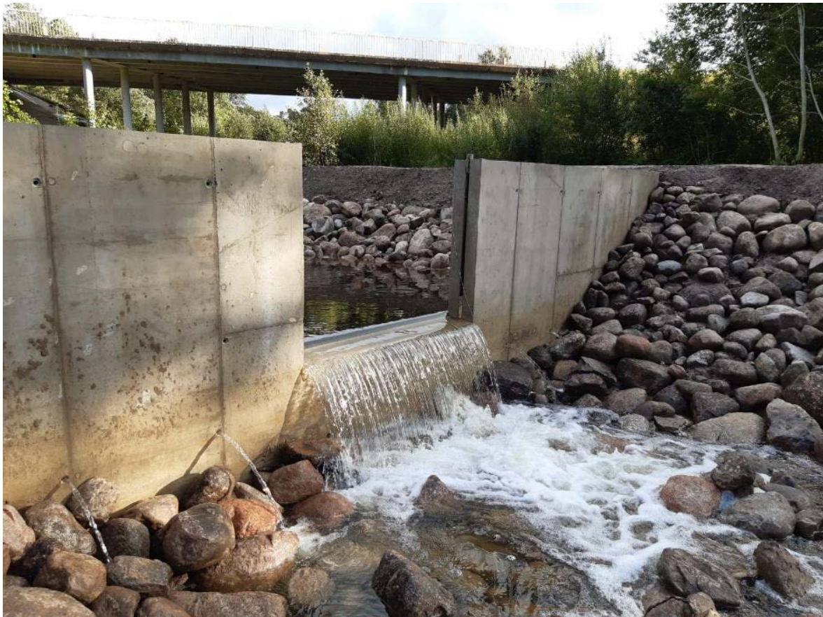
Figure 24. The fish pass site after construction in September 2020 (Photo credit: Kaspars Abersons).
