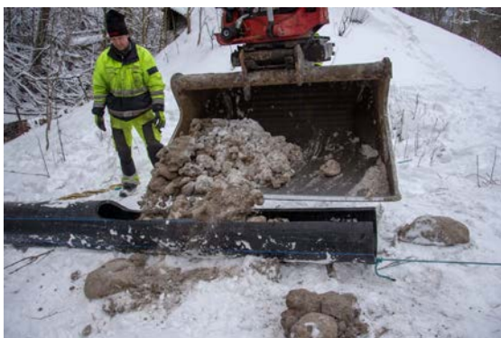
Figure 48. The deployment of gravel on stretch 3 was carried out with an excavator and a specially adapted pipe. Photo credit: John Kärki.
