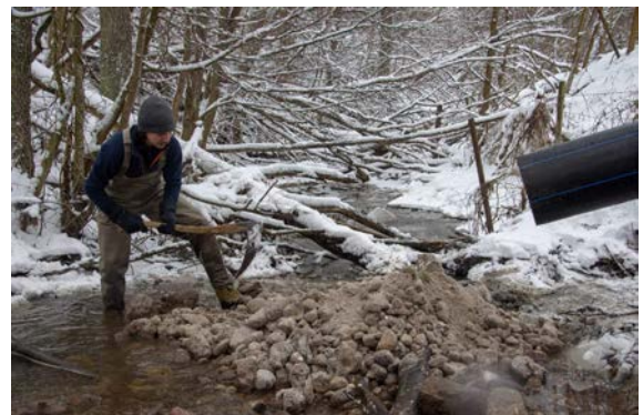
Figure 49. When the gravel had been added to the watercourse, it was distributed by hand. Photo credit: John Kärki.
