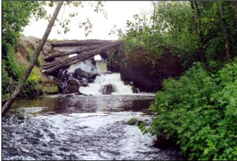
Figure 4.26. The Solka River, dam
