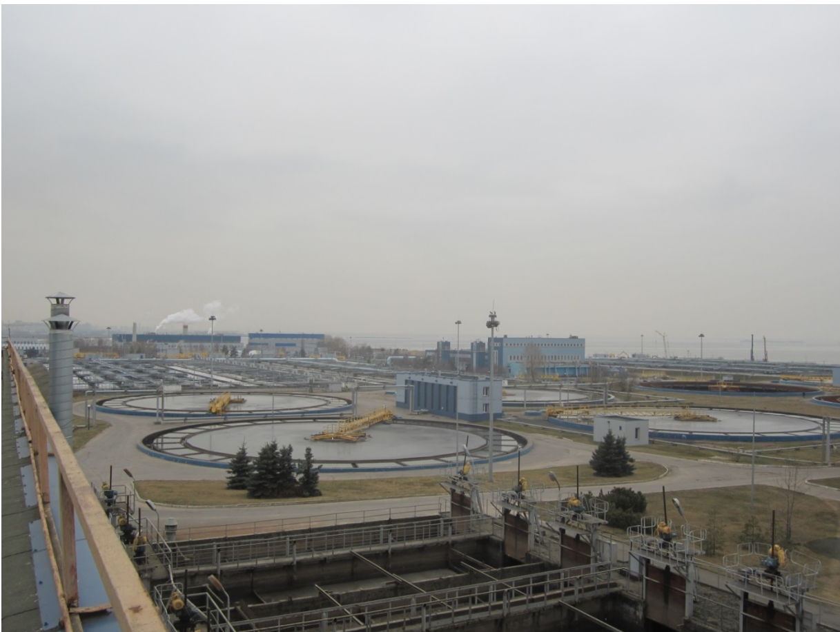
Figure 1. Picture of the Central Wastewater Treatment Plant of Vodokanal of St.Petersburg
