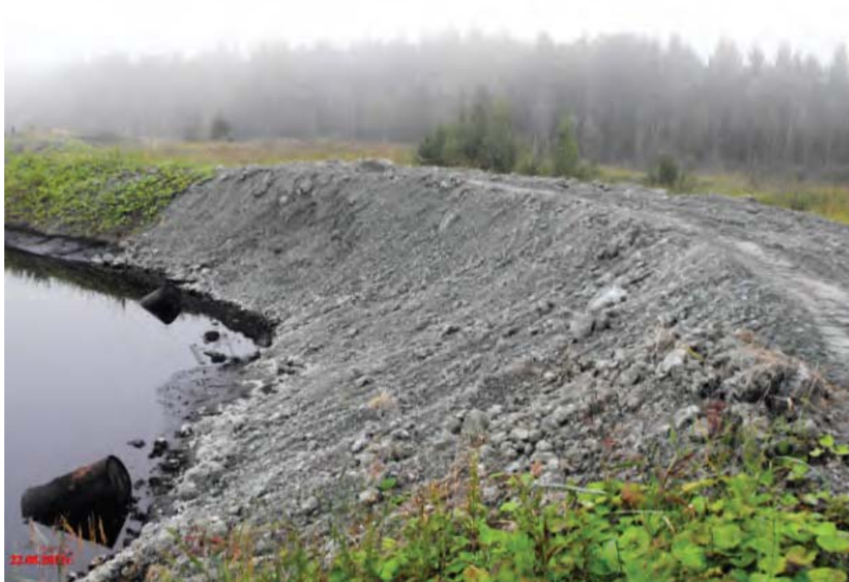
Figure 6 – The results of maintenance of flood-wall of foundation pit № 68
