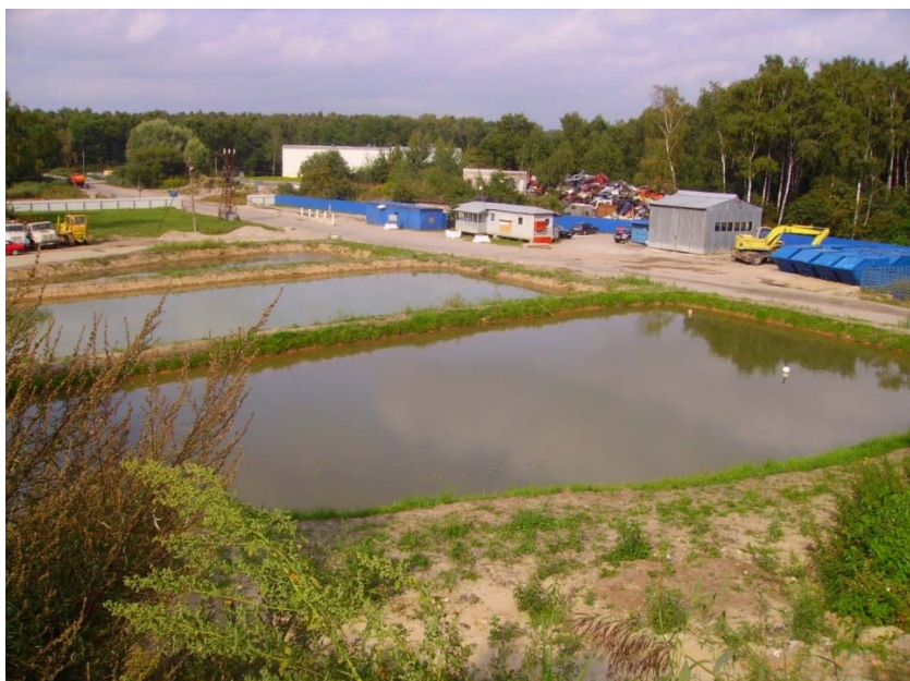
Figure 34 – The pilot facilities for collection and treatment of filtration water at the landfill of hazardous wastes of Kaliningrad
