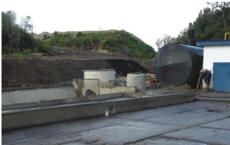
Figure 33 – Suction sumps at the Landfill of hazardous wastes of Kaliningrad
